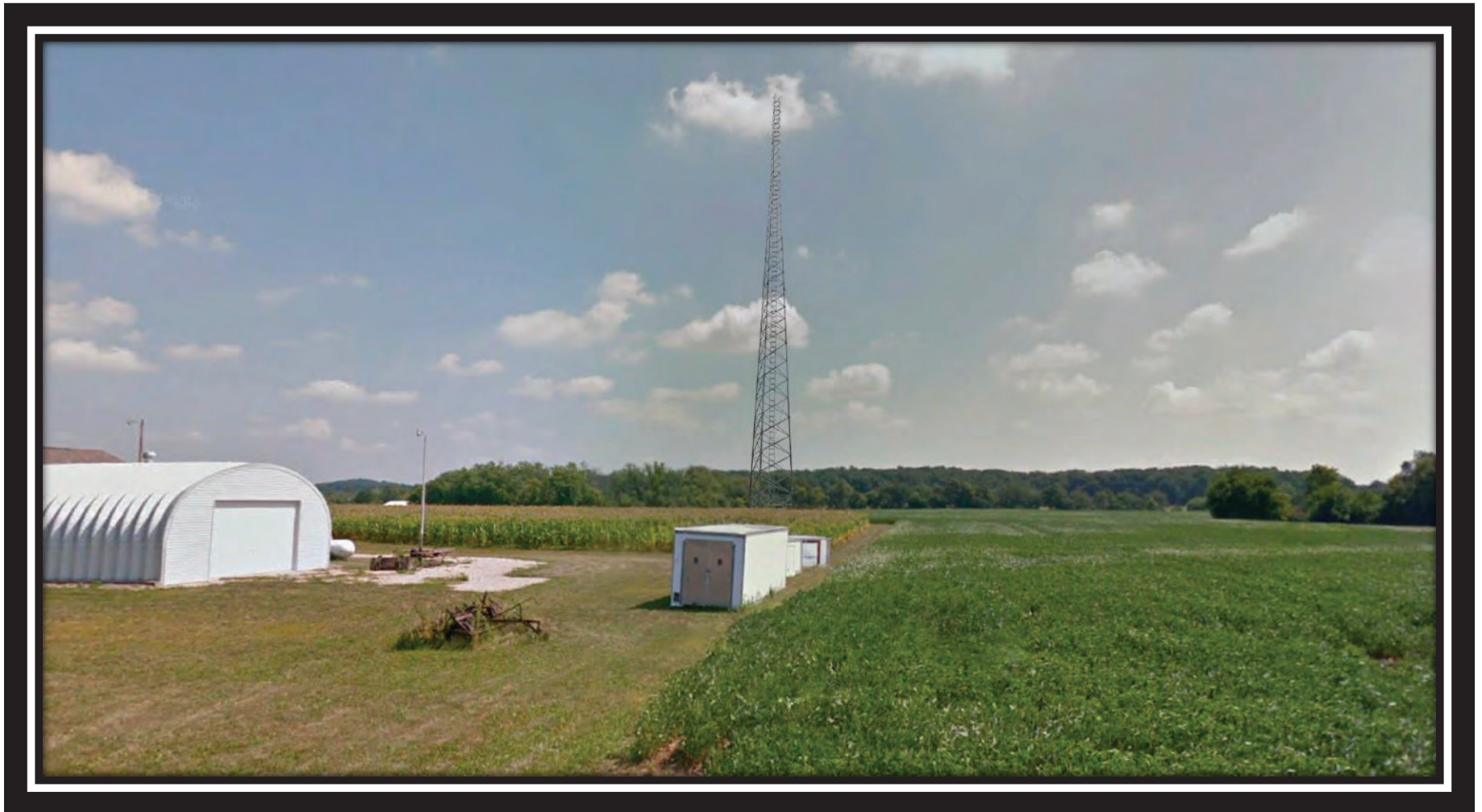
Photo Location Directly West – {After}
