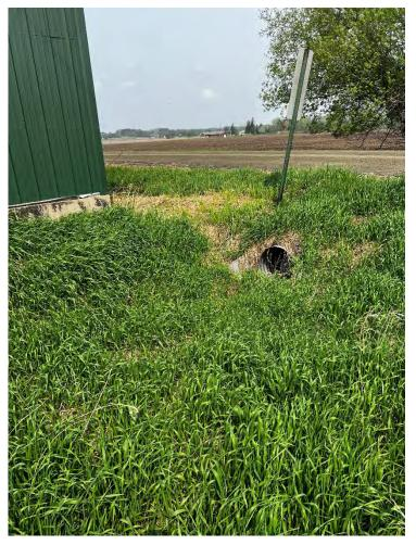
Photo 1: Culvert crossing under road adjacent to farm field. This ditch and culvert is most likely catching any road runoff adjacent to the farm field.
