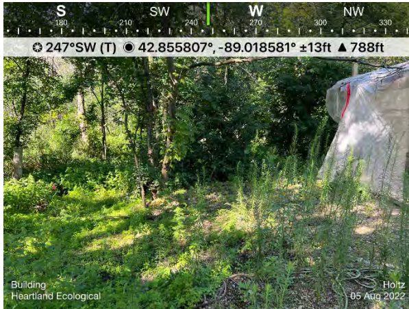
Photo # 7 Photo of unfinished building on property- west view
