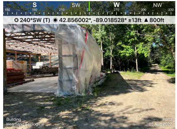
Photo # 4 Photo of unfinished building on property- west view
