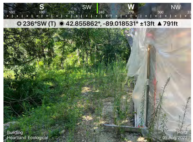
Photo # 6 Photo of unfinished building on property- southwest corner
