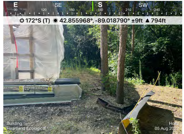
Photo # 2 Photo of unfinished building on property- south view
