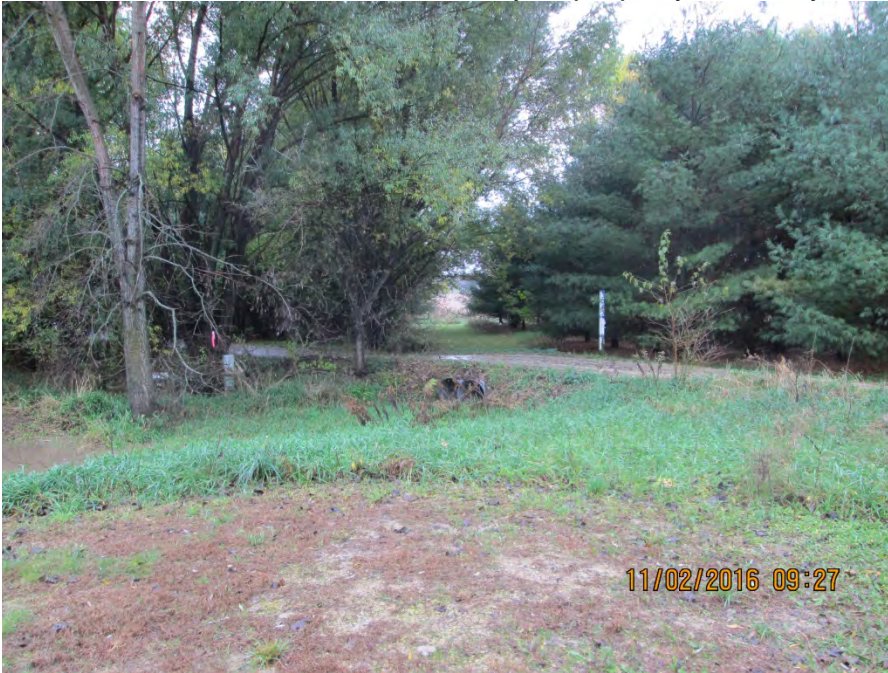
Picture shows the culverts under Payne property driveway
