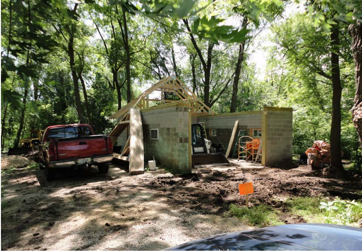
June 26, 2018-new trusses and issued stop work order
