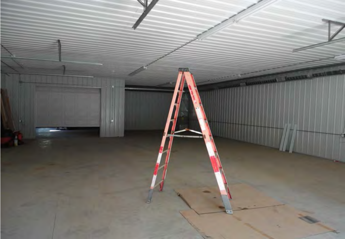
Inside of building – heated
