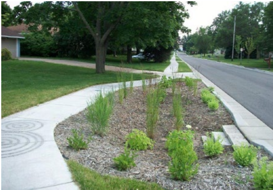
Example of vegetated swale in Maplewood
