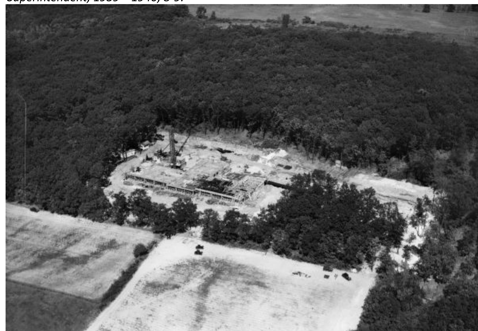
Lake View Sanatorium under construction, 1929 (source: Wisconsin State Historical Society Archives, 35103, by Arthur M. Vinje).
