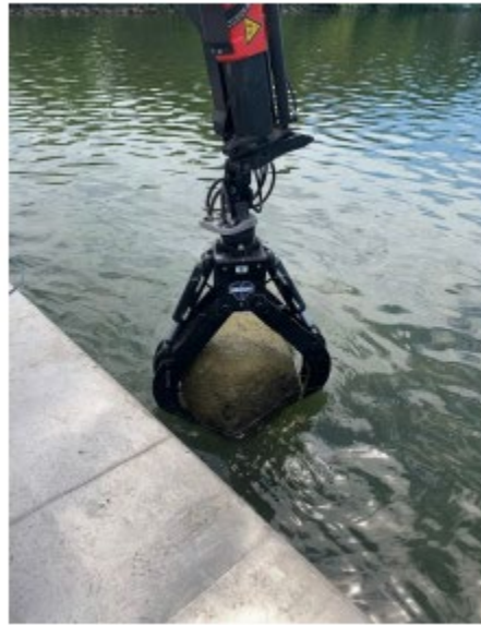
Dredge equipment removes sediment and obstructions from the riverbed.
