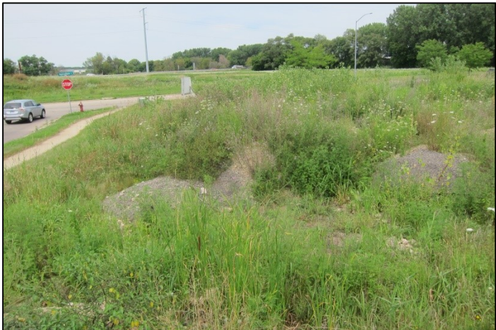
Typical fill found on several lots
