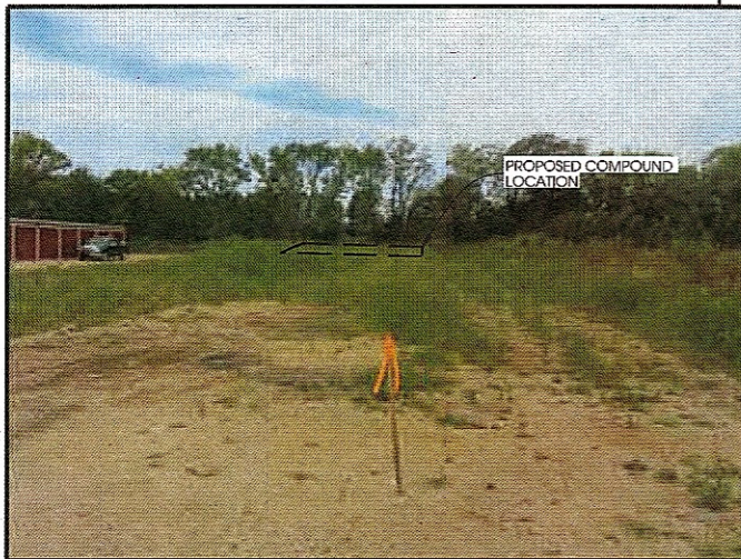
SITE OVERVIEW (LOOKING WEST)
