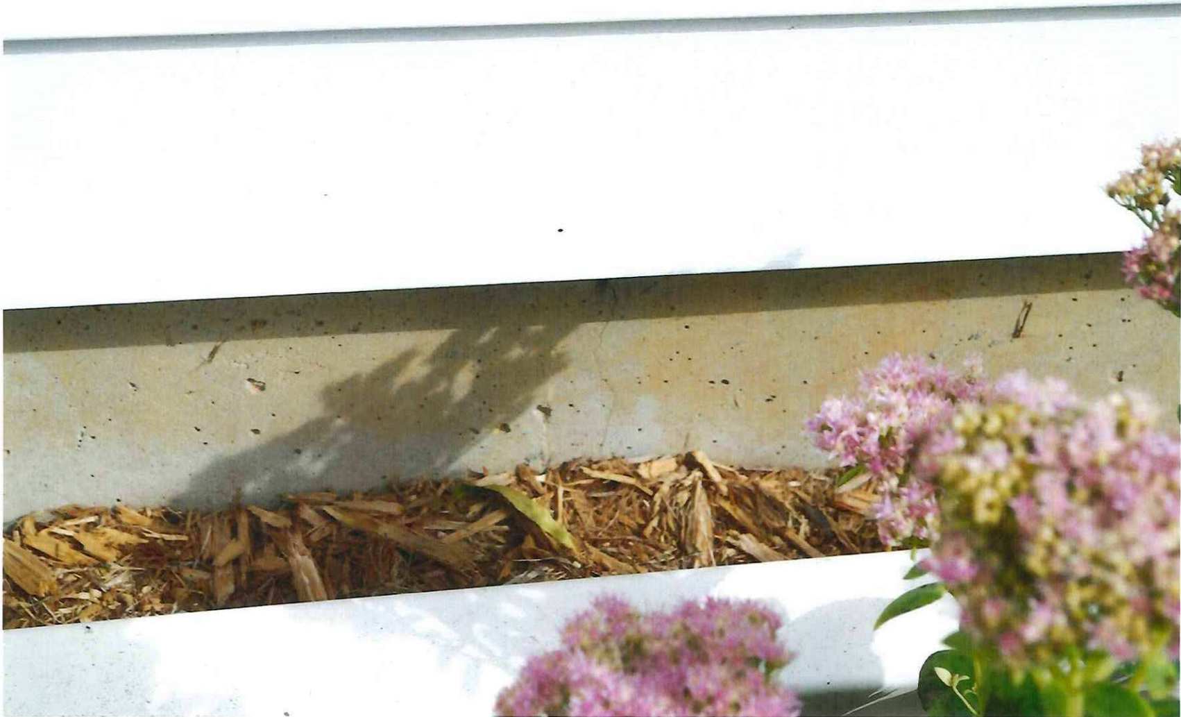
Photo from Pre-blast Survey in 2014
