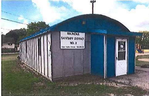
North façade (Front facing Thurber)
