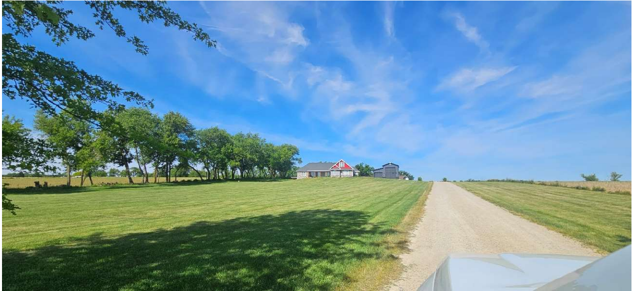
Exhibit E: Existing accessory building (view from driveway) -Shown at public meeting
