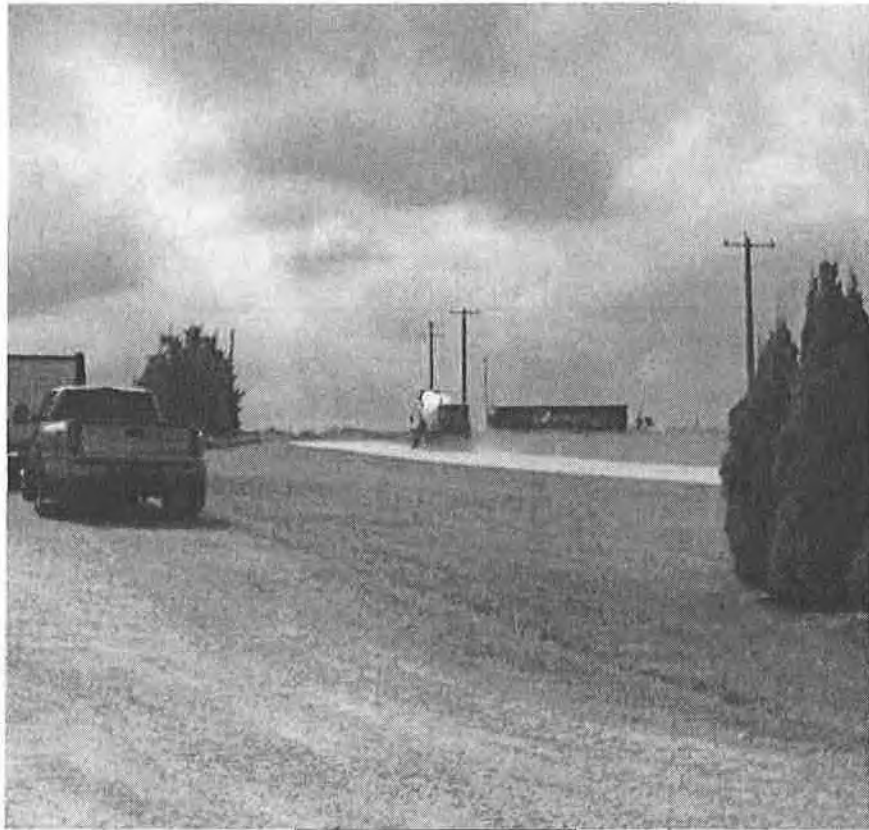
Concrete Truck Exiting
