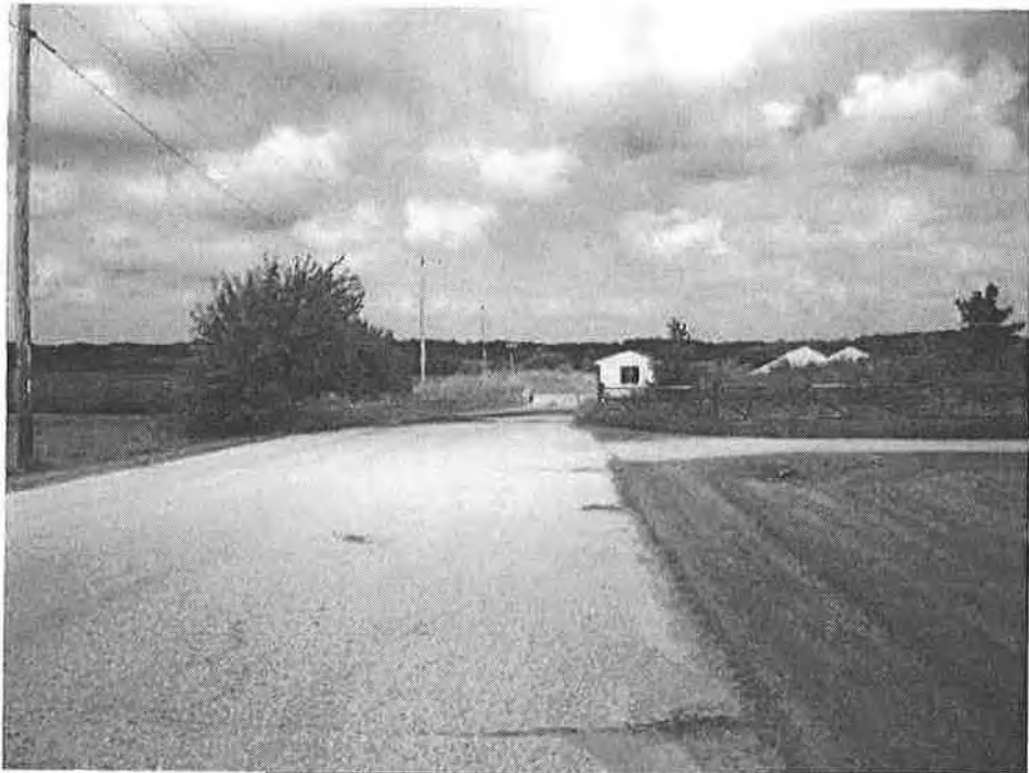
Gravel Pit and Concrete Plant Access
