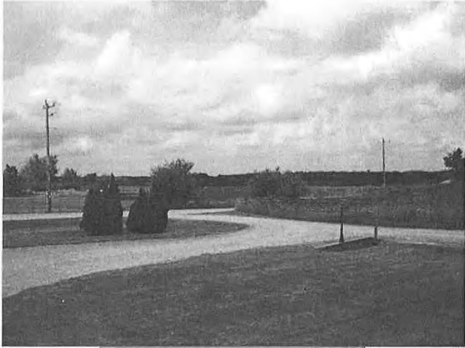
Subject Driveway and Concrete Plant Access
