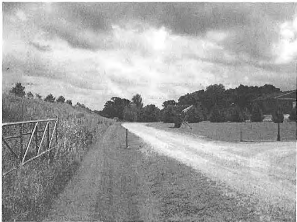
Access Drive and Berm
