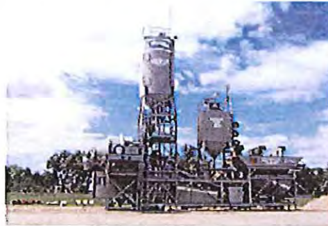
Portable concrete batch plant
