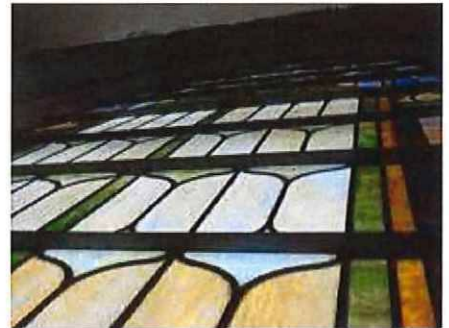
6. Windows not bowing
