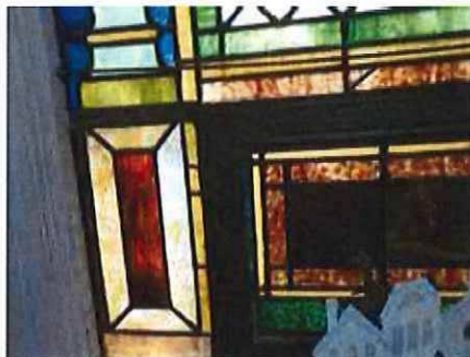
8. New aluminum ventilator
