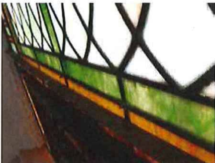
7. Detached reinforcement bar above new ventilator
