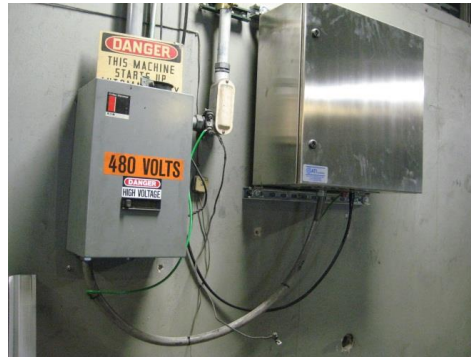
Photo 10: East Penthouse Microwave Enclosure
