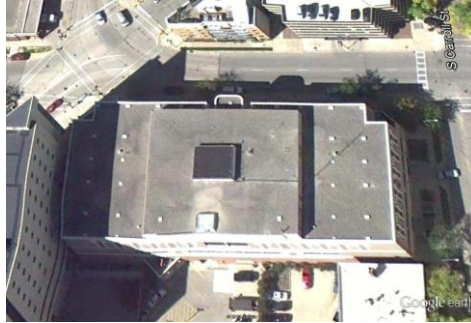
Figure 1 - Aerial View of Building
