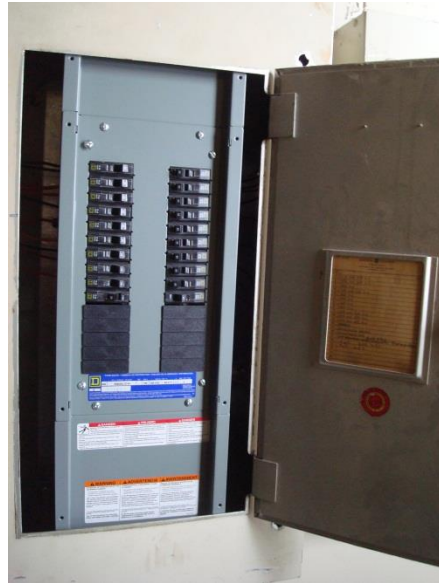
Panel LP6 2 (Sixth Floor East)
