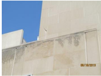
Photo 13: Parapet damage
