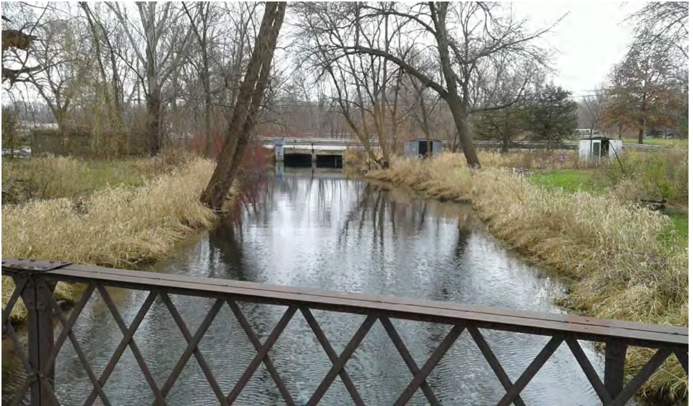
Photograph PP-05; facing west.
