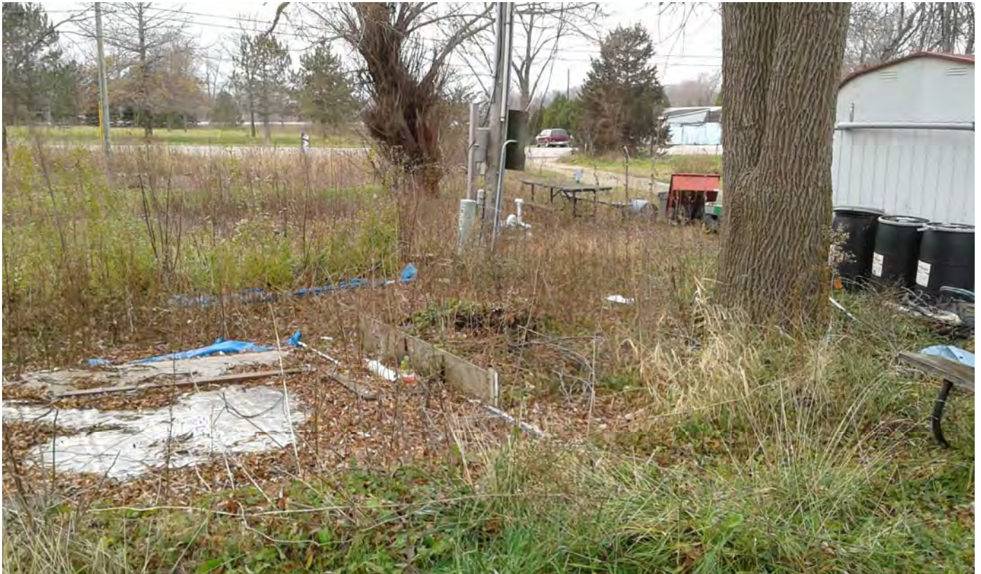
Photograph PP-12; facing northwest.
