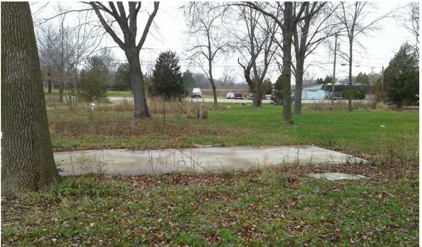
Photograph PP-02; facing west.
