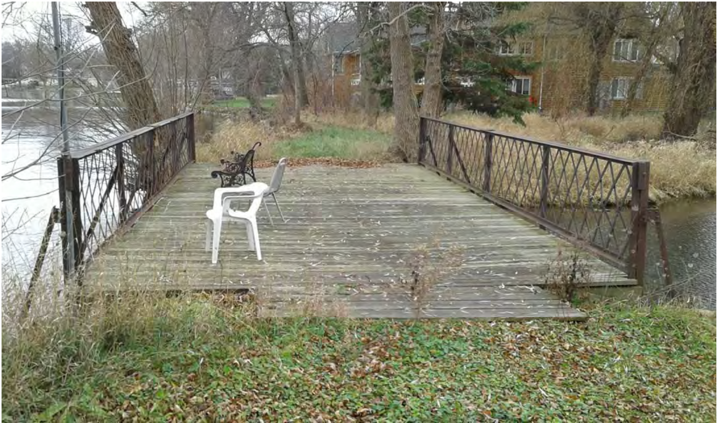
Photograph PP-11; facing south.
