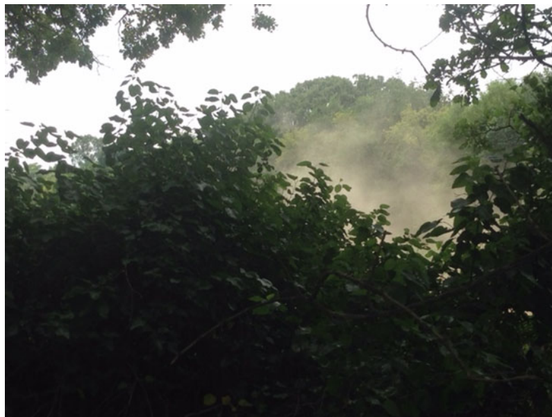
Image 2 – Dust cloud generated during quarry material removal on 8/6/2021 12:50 pm
