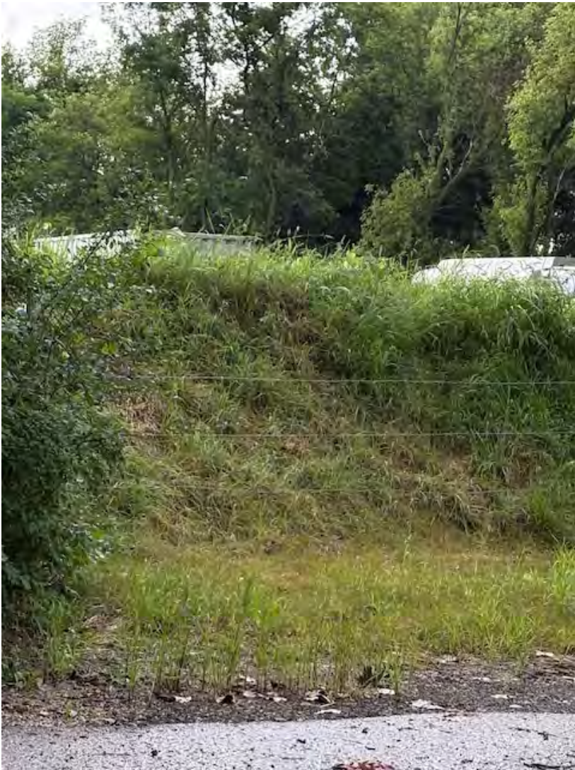
August 18, 2025 - North gate berm
