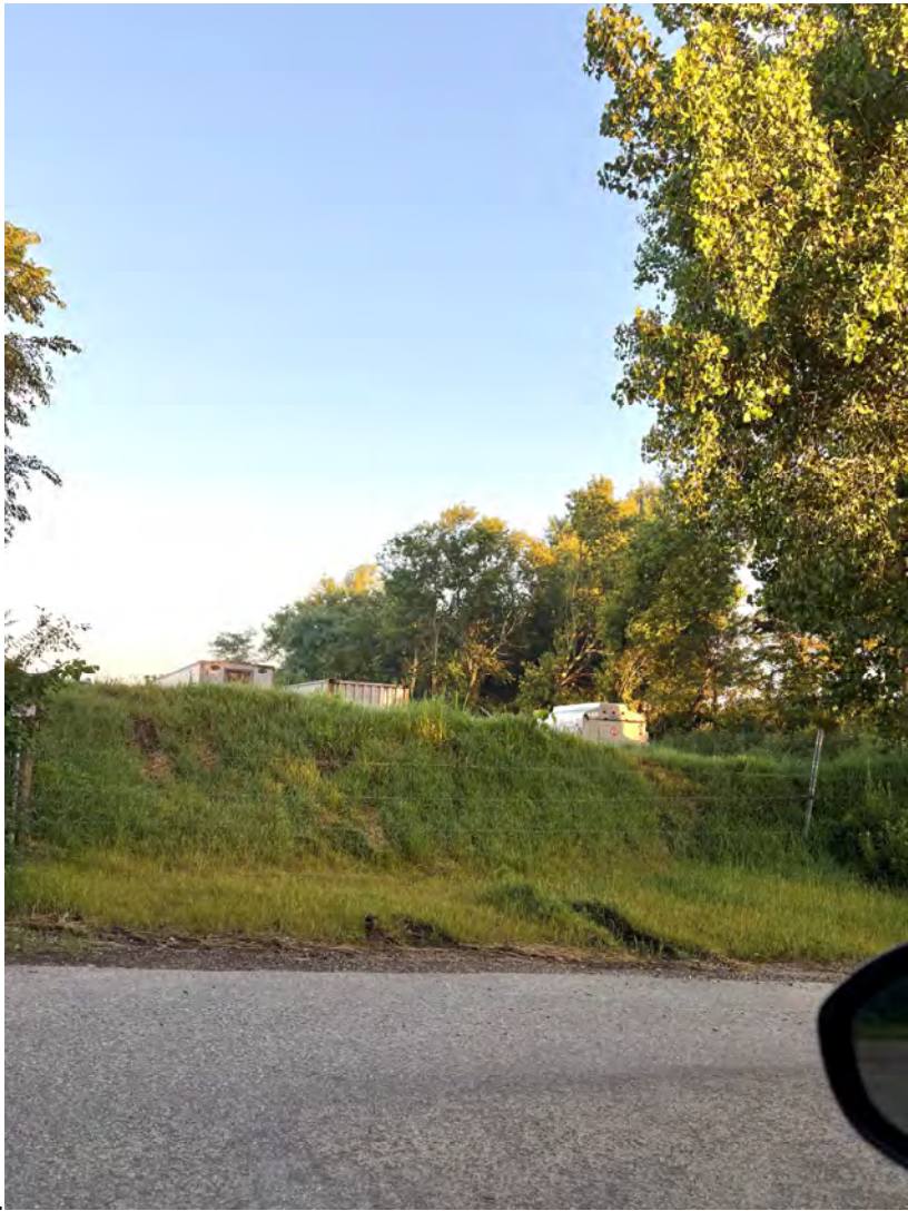
August 18, 2025 - North gate berm
