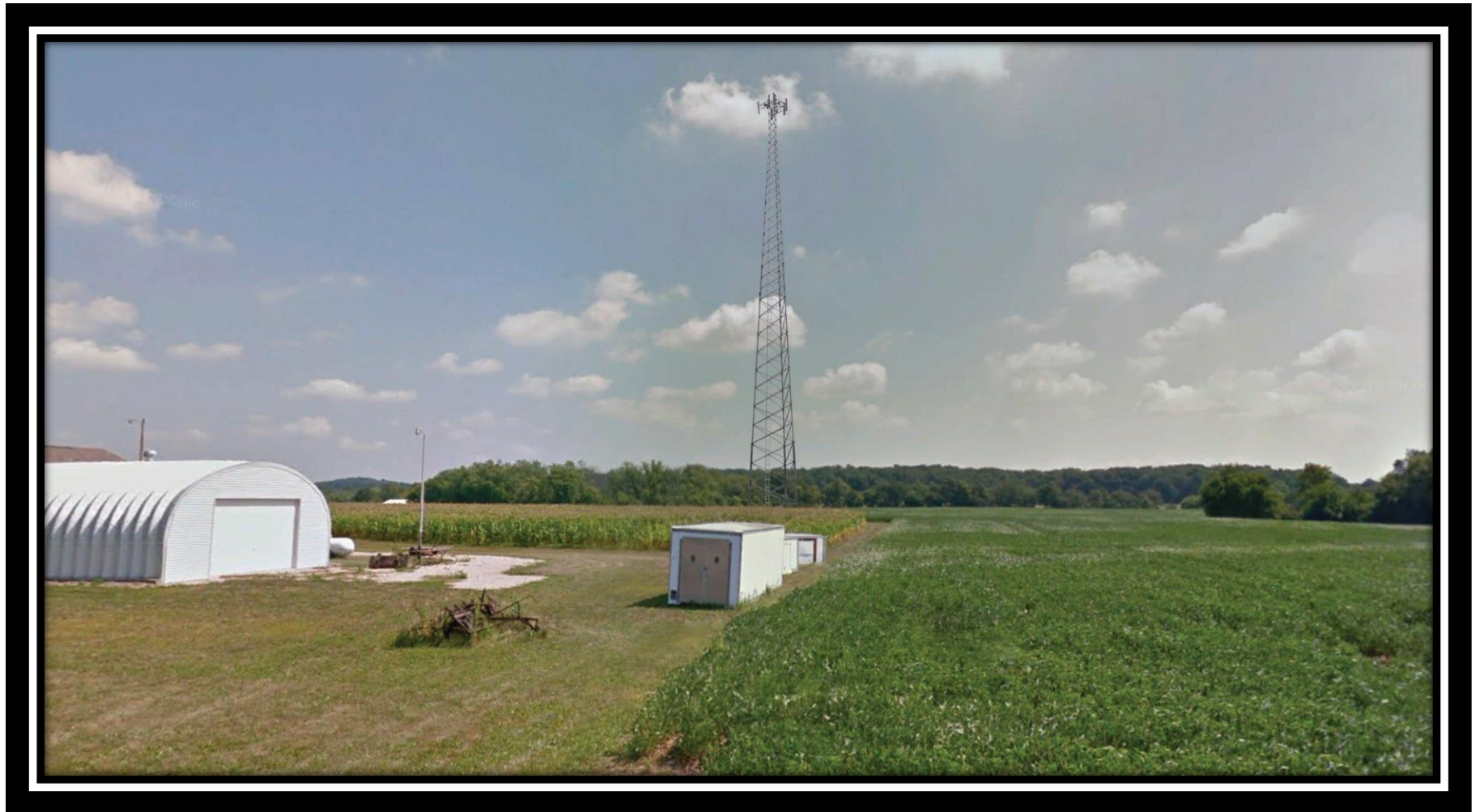
Photo Location Directly West - {After}
