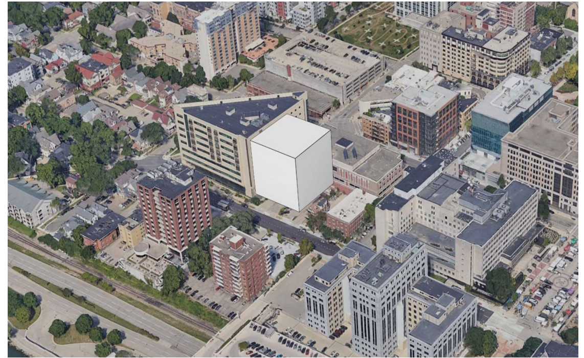
South Tower Addition & Public Safety Building Renovation
