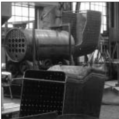
Fig. 5: Construction of the boilers.
