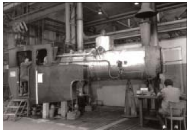
Fig. 2: Test stand for the new light oil firing. The boiler is provisionally insulated. The cab is a mock-up.
