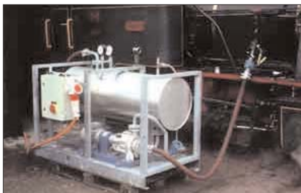
Fig. 9: Two flexible hoses connect the boiler to the preheating device. Note that the hoses can only be disconnected if both ball valves are shut. This ensures that the preheating device cannot be disconnected under pressure.
