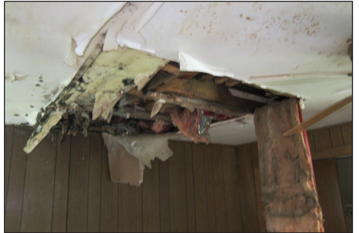
Living rooms and water damaged ceiling below upper bathroom
