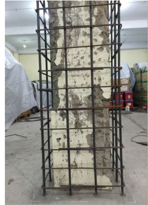
INCREASE COLUMN PLAN DIMENSIONS
