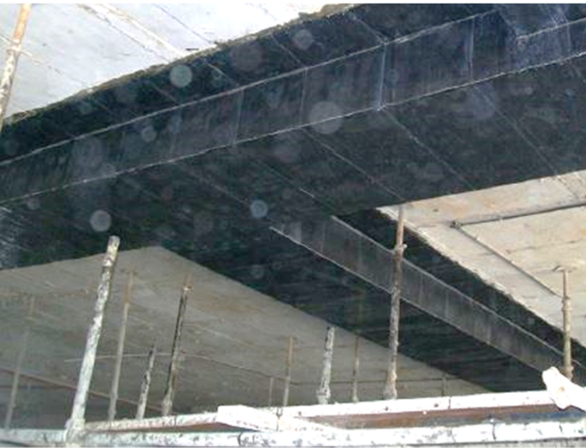
CARBON FIBER-REINFORCED POLYMERS (CFRP) WRAP
