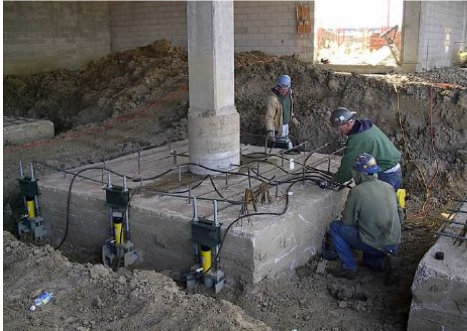
UNDERPINNING FOUNDATION
