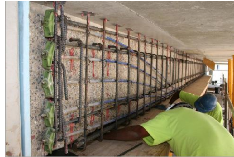
EXTERNAL POST- TENSIONING APPLICATION
