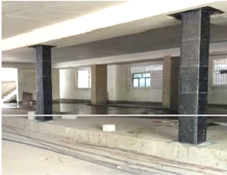
CARBON FIBER-REINFORCED POLYMERS (CFRP) WRAP
