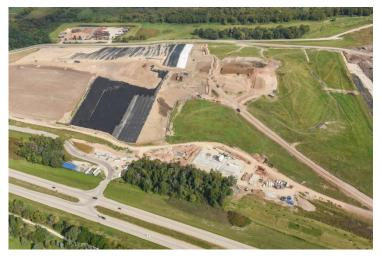
Construction of approximately 34 acres of final cover was completed on inactive phases of the Rodefeld Landfill. The final cover system includes layers of compacted soil, a geosynthetic clay liner, and plastic geomembrane which minimize intrusion of water into the landfill and the amount of landfill gas that is released to the atmosphere. This major capping project will reduce the amount of leachate that is generated by the landfill and increase efficiency of the landfill gas collection system
