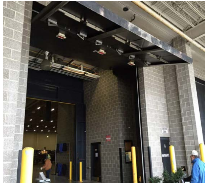
The Coliseum's high-speed door prevents significant heat loss, reducing gas usage and providing monetary savings for Dane County.
