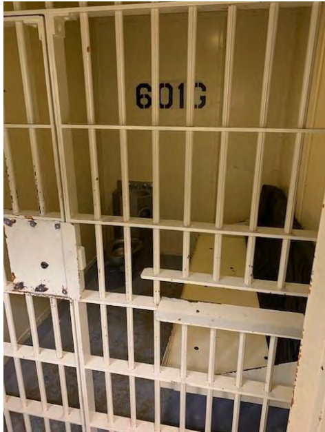
Existing CCB Cell Blocks
