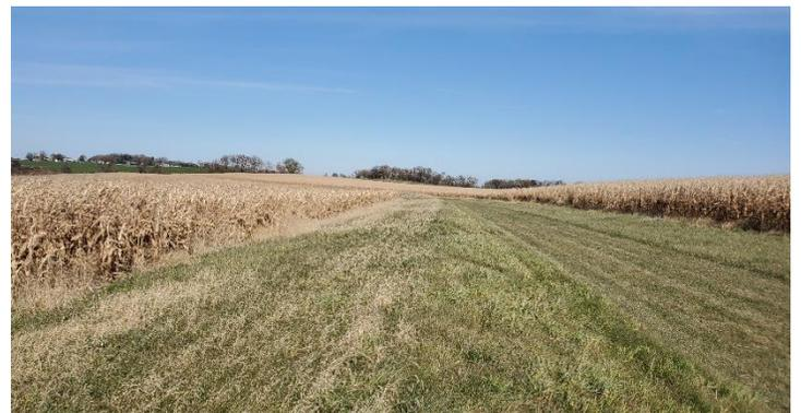
Water and sediment control structure (top photo). Diversion directing water into the water and sediment control structure (bottom photo).
