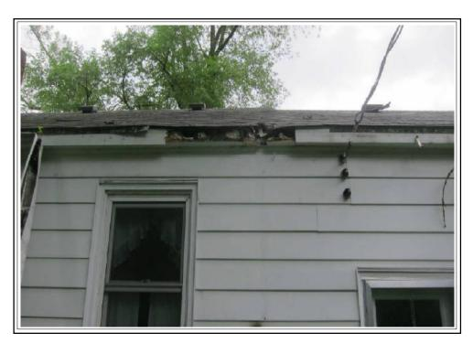
Rear roofline where electrical mast broke off eave and side of dwelling.
