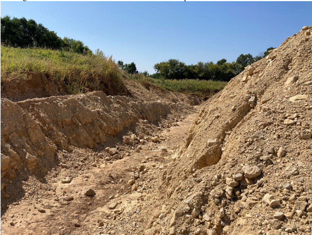
Looking west to where the stormwater drains into the sand portion of the site
