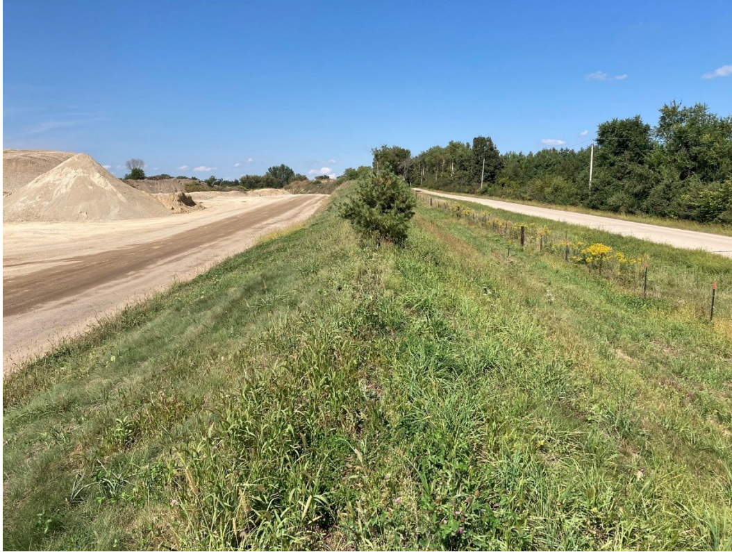
Center Road berm and plantings, September 11, 2025 photos
