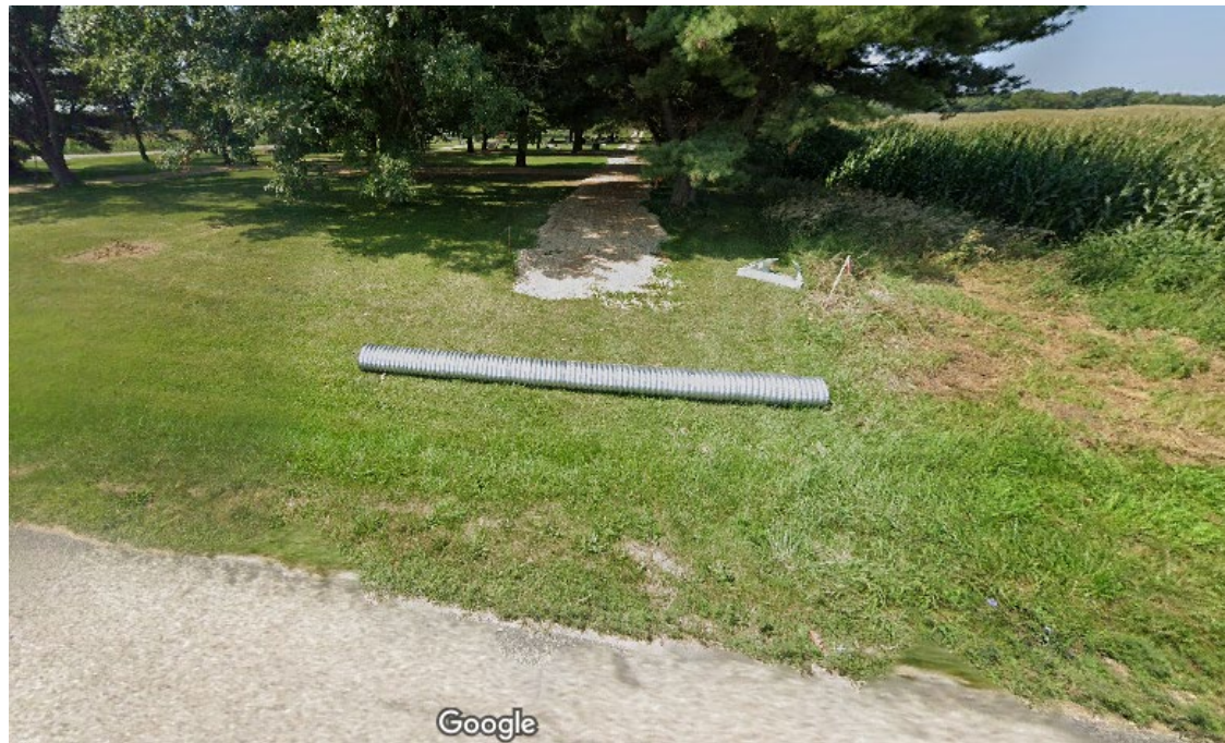
Street view August 2023 – new culvert for cemetery
