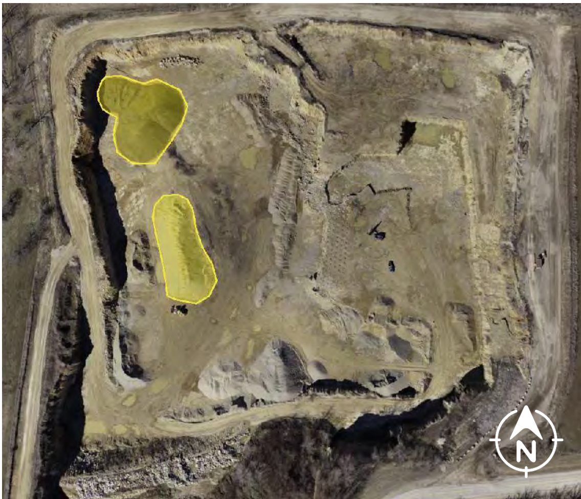
Figure 2: Map showing the general locations of raw material stockpiles that could interact with stormwater. Portable crushing equipment is also temporarily operating within this space.
