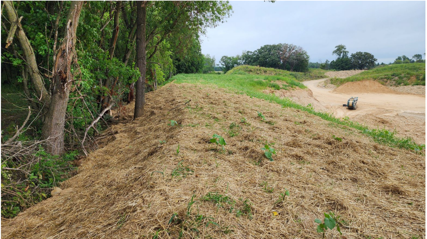
Looking north along the westerly property line.
