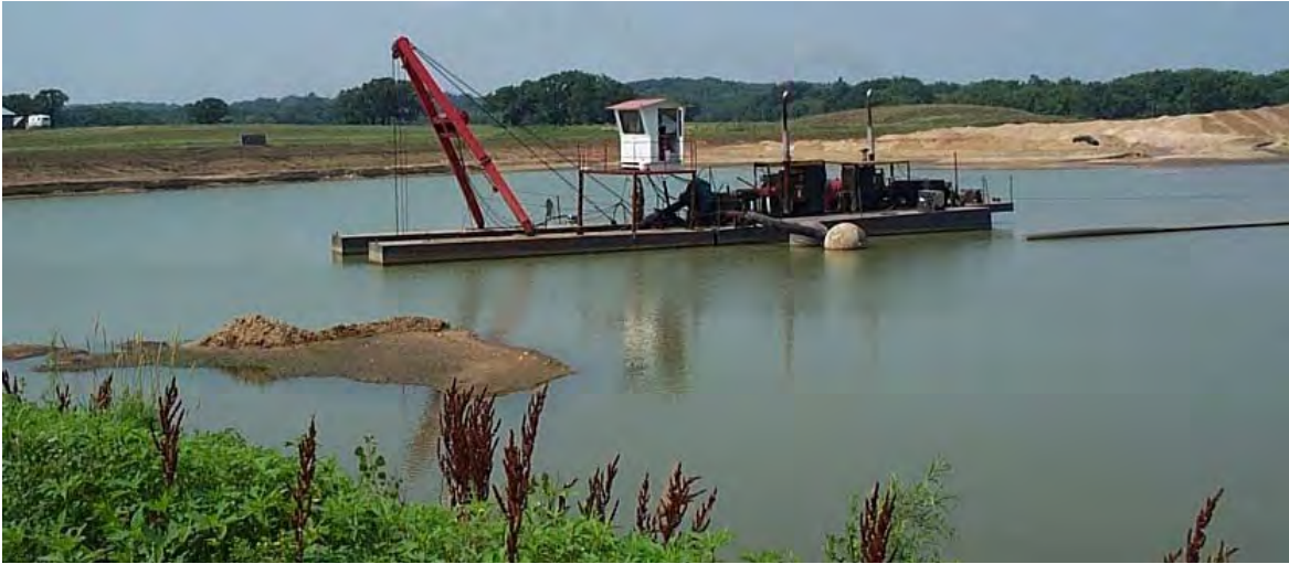
Figure 5. Donovan pit mining with a hydraulic dredge.
