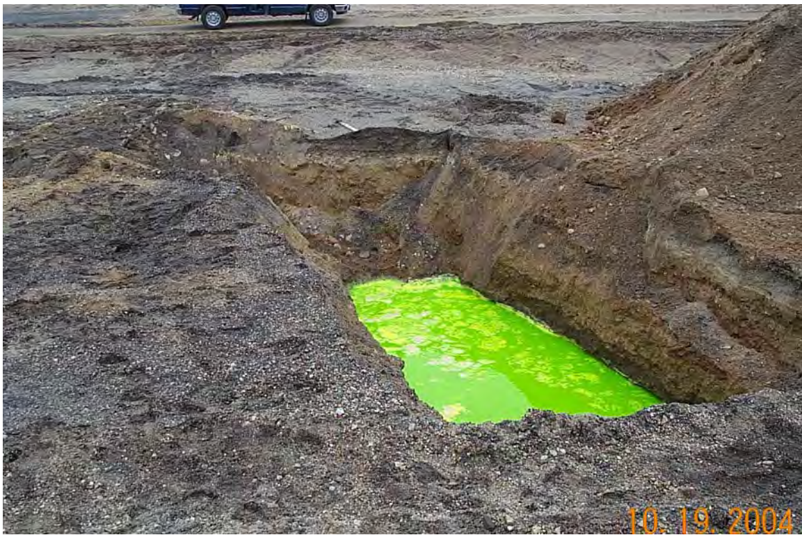
Figure 8.6. Trench 1, dye injection point.
