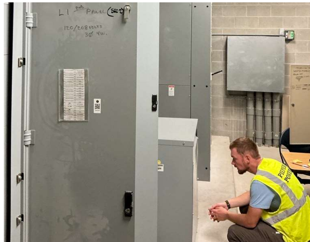
Pictured above is an electrical evaluation
