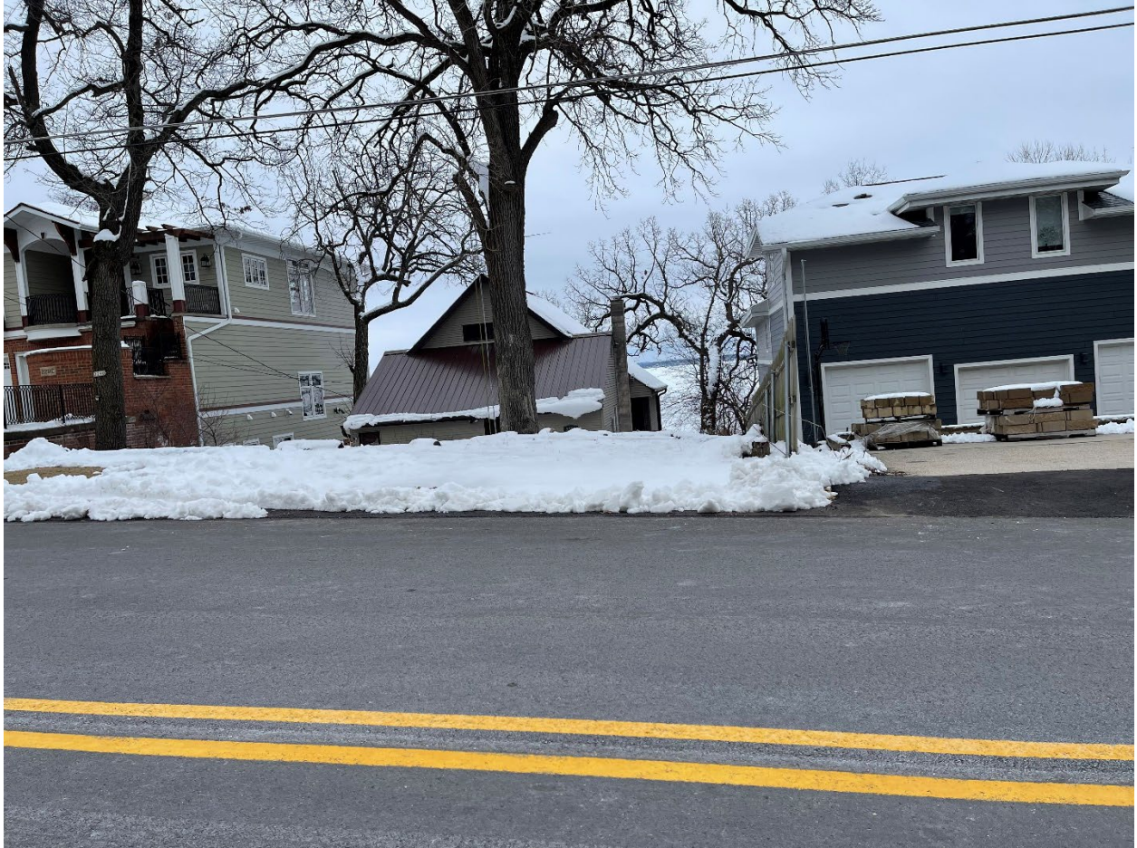
Parking area ill defined.
