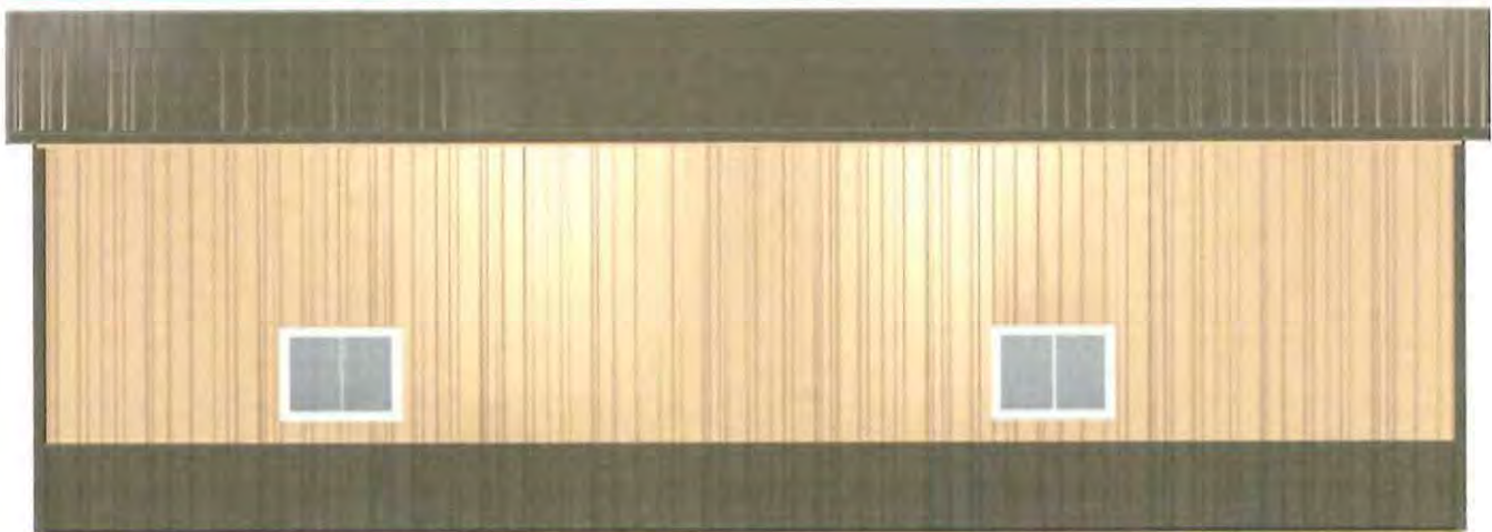
South Side Wall 1 on Building 1
