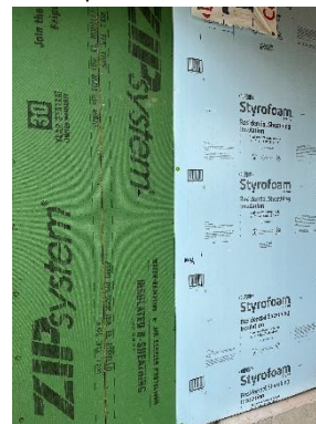
Second Townhome Insulation
