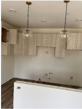
Townhome Unit Interior
