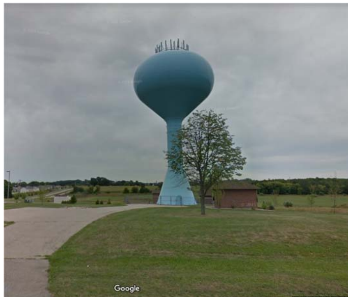
Water Tower as seen from Holscher Road (Source: Google Maps)
