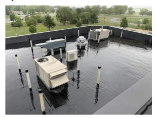
Based on the age of the building, the existing roof system would be within the limits of a typical 20- or 30-year warranty period. Given the condition of the roof, it is our recommendation that the existing roof has at least 10 years of useful life remaining.
