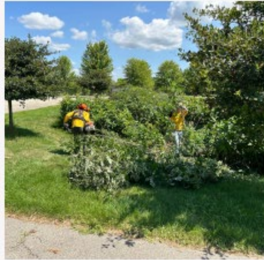
The OFS crew cleared woody vegetation from the bioretention basins at Babcock County Park.
