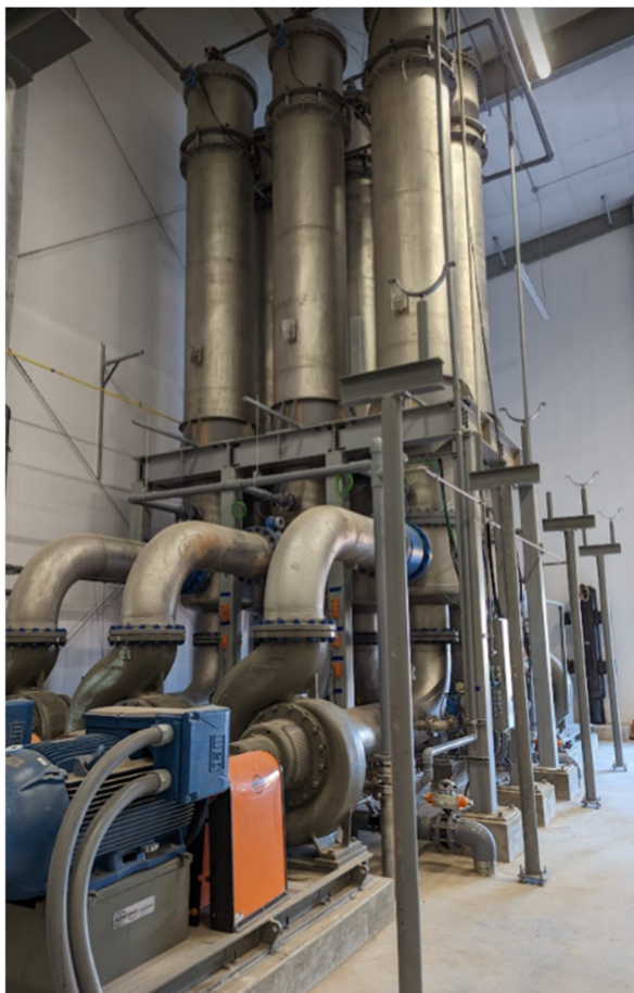
Figure 8: Stainless Steel Ultrafiltration System for Digested Dairy Manure
