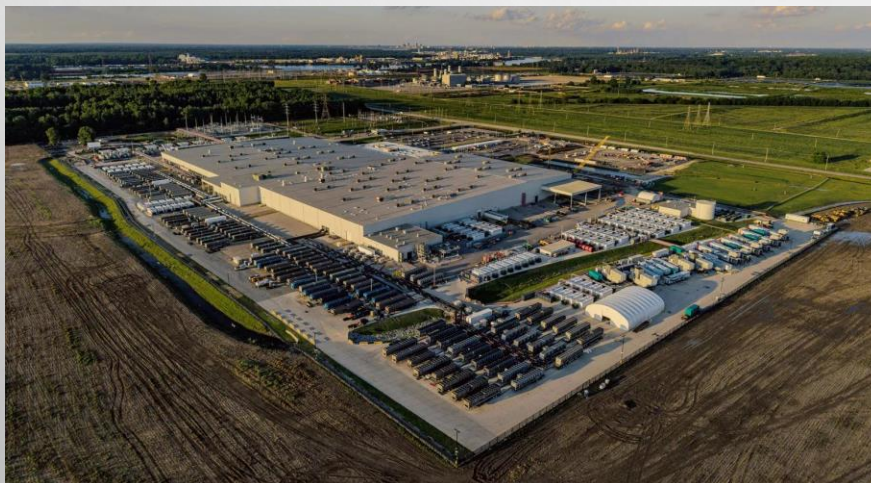
The xAI Colossus data center in Memphis, Tennessee, May 2025. Source: Stephen Voss/Redux
