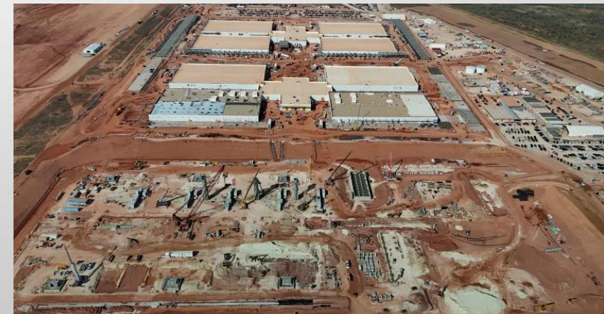
Aerial view Crusoe's Abilene, TX data center under construction. Source: Crusoe
