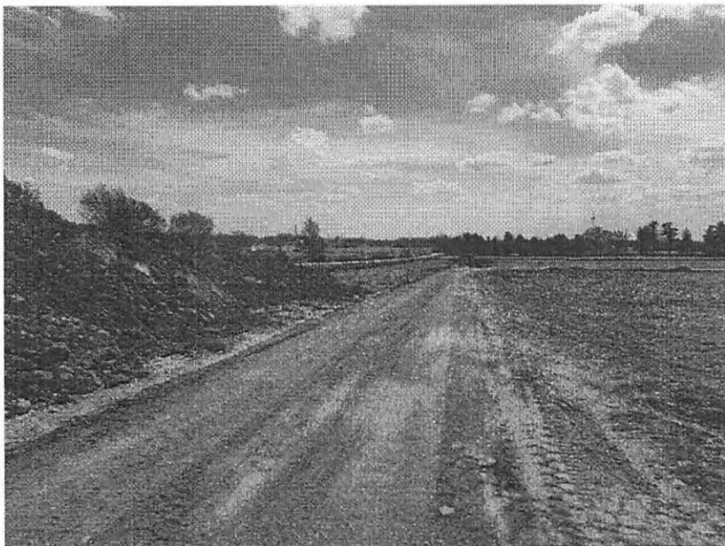
Looking south along Center Rd.
