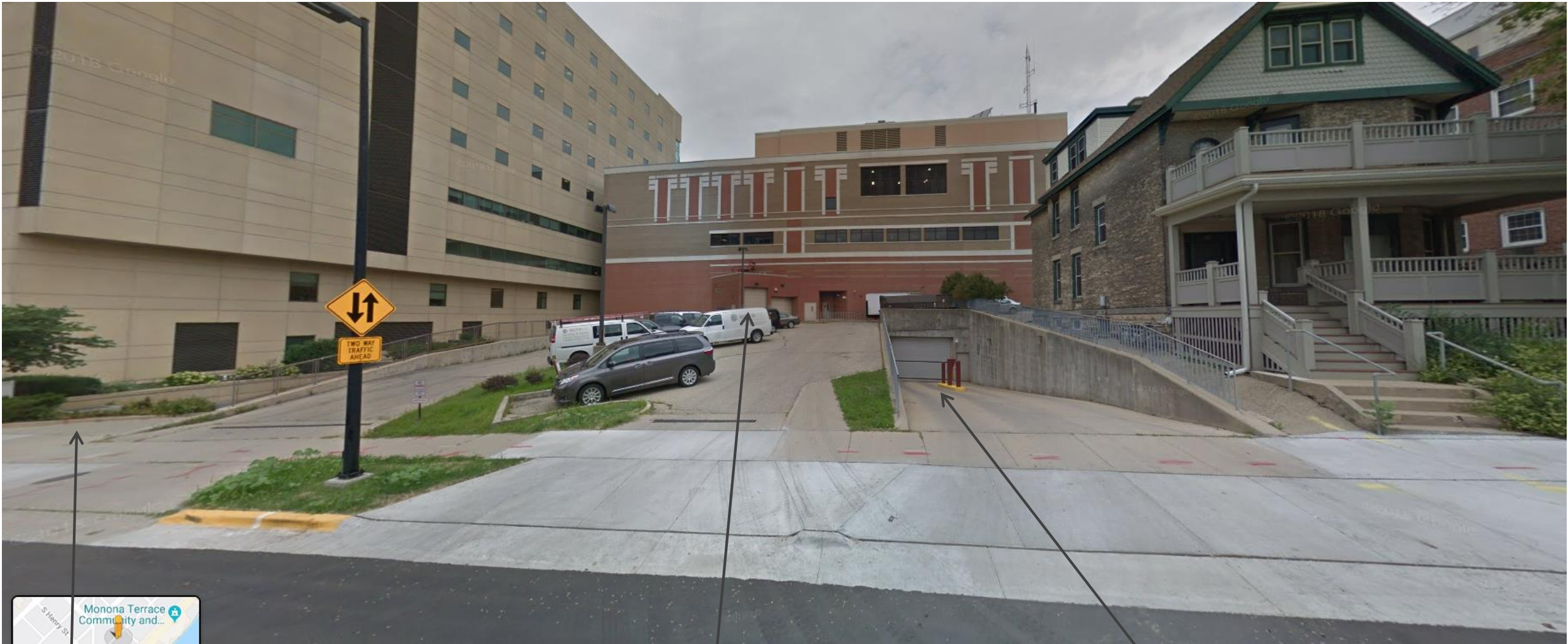
Courthouse garage entrance
